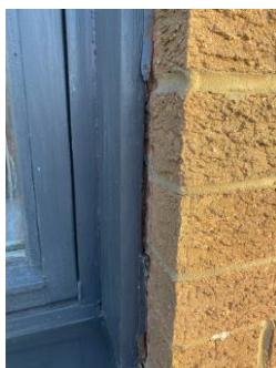
Sealant missing
