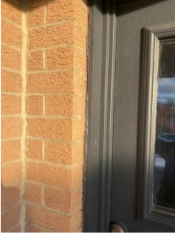
Sealant missing
