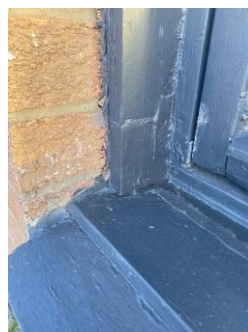
Spliced timber repair
