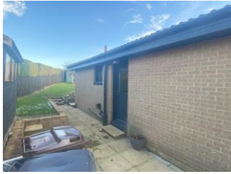
Timber fascia boards
