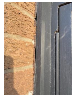
Sealant missing
