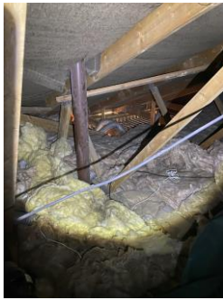
Cut felt for service penetration
