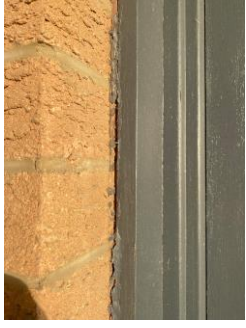
Sealant missing
