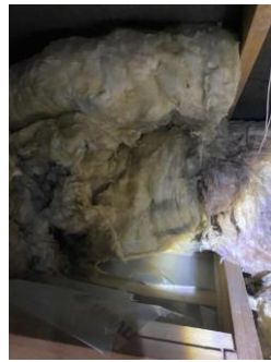
Displaced insulation
