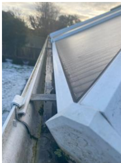
Blocked gutter
