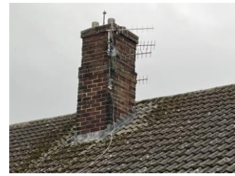
Areas of repointing
