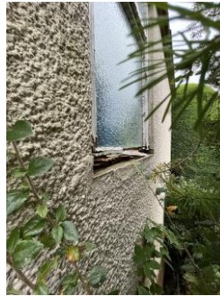
Decayed timber window
