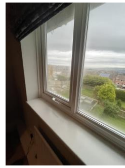
Rear elevation window
