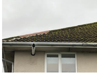
Hip tiles have been replaced
