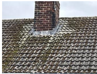
Lead work appears satisfactory
