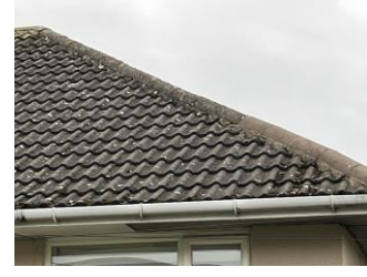
Hip tiles have been replaced
