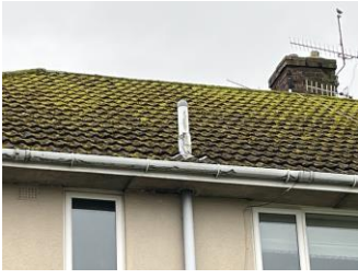
Repaired soil stack above roof line
