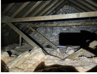
Displaced insulation
