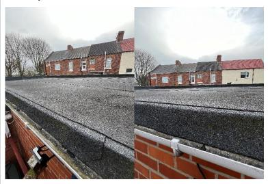
The felt roof appeared out of level, arching from front to back, this could have been caused by water ingress and the roof decking absorbing moisture. A roofing felt lifespan is between 10-20 years. The felt roof may be repaired to prevent water ingress to the garage roof timbers. An approved flat roofing contractor should be appointed to assess repair costs against recovering the entire roof covering.
