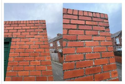
The masonry has diagonal cracking to the front elevation. Diagonal cracking can indicate structural movement. It is advisable to obtain further advice from a Structural Engineer regarding the structural movement. The Engineer may suggest monitoring or repair works to the structure.
