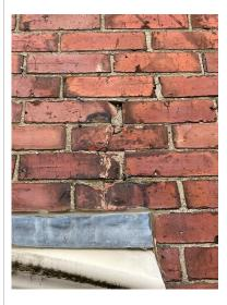
There is vertical cracking to the masonry above the front bay window opening, the cracking extends to several courses of the masonry. It cannot be determined from the survey the cause of this but may be due to the installation of the new window
