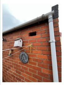
The brickwork will need to be replaced to prevent vermin entry/cold bridging and possible brickwork instability.
