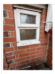
There are sections of the window that are decayed and rotten, and the extent of which is unknown. Sections of timber rot can be removed and spliced with new timbers. I would recommend obtaining estimates of works from competent contractors before the exchange of contracts as it may be more economical to replace the window rather than carrying out repairs.
