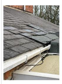
There was no ventilation provision within the kitchen roof. Timber roof structures require cross ventilation to ensure the timber remains free from rot and decay. Ventilation channels should be provided.
