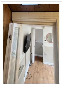
The conservatory is not separated by external doors to the main property. The conservatory may now require building regulation approval and checks should be made with the local authority building control. The conservatory must be separated with external doors to be exempt from building control approval.
