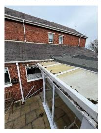
The roof covering is a mixture of Upvc panels, and a flat roof felt. The joints should be checked to ensure moisture does not enter the building around joints.
