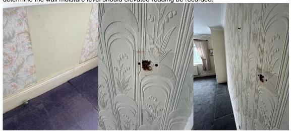
There were several holes to the plaster and partition walls. The wallpaper will have to be removed in this area for the plaster board repair to be carried out. The hole may be filled with a back board and filled and sanded over.
