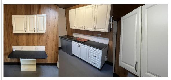
Several cupboard and drawer fronts require realignment as this can cause the front of the unit to snap away from the draw shelf unit during use.
