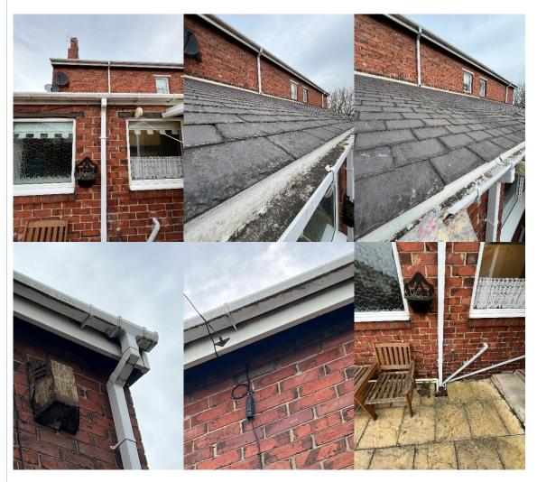
The guttering and downspouts appeared to have moss and algae growth. These should be cleaned at the first opportunity to prevent further growth which may lead to seals and gaskets becoming damaged.
