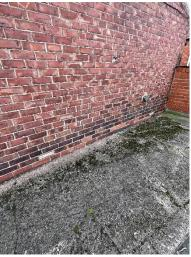
The air vents to the side elevation have been blocked/filled with mortar pointing. Air vents prevent humidity and condensation forming beneath a suspended floor. It is advisable to install clear these air vents at the earliest opportunity. The timber floor joists should be checked to ensure rot and timber decay hasn't started.
