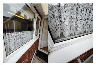
The window frame has external glazing beading which is no longer used in a modern window design. The external beading and double-glazed units can be removed externally. It is advisable to make enquires with the proposed property insurance company, as external glazed beading may be an exclusion from an insurance policy. I would recommend replacing the window frames for property security.
