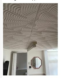
The ceiling is covered with polystyrene tiles. Polystyrene ceiling tiles and coving can be a major fire risk. An out-of-control house fire can produce poisonous gaseous fumes and the plastic in the polystyrene can drip and burn your skin as it falls. I would recommend replacing all polystyrene tiles with a plasterboard ceiling.
