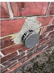
There are redundant gas flues to the front and side elevations. The openings appear to have been filled internally. Openings in the masonry wall can allow moisture to enter the cavity unnecessary causing damp to the internal walls. These should be removed and the opening closed by a suitably competent person.
