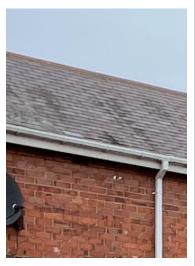
The flat roof conservatory construction abuts the rear mono pith roof and the joint has been formed by inserting the roof felt under the original slate roof, this has displace the seating of these slates and could allow moisture to enter the roof structure.
