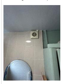
The extractor fan did not operate when in the on position. An extractor that is not operating correctly can allow excess moisture to build up within the air and circulate around the property structure. Once the warm moisture laden air, meets a cold surface, saturation of surface capillaries can occur leading to mould spores. Should the extractor not operate correctly when in use, a suitably qualified and experienced person should be appointed to provide and install a suitable extractor.
