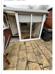
Glazing that building occupants are likely to come into contact with must meet one of three requirements: If broken upon impact it will break in a way that will not injure anyone, resist impact without breaking or be shielded or protected from impact. The full height glazing units did not have any Kite marking visible and should be checked for their suitability in regard to glazing in critical areas
