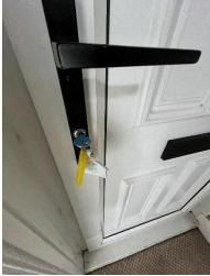
The front door does not close into the door casing correctly. The door appears to have dropped and catches at the threshold, or the original installation was out of alignment (plumb) from the door to the casing. The doors may need to be replaced or adjusted by a competent person.
