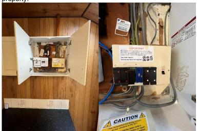
The fuse box is dated, and it is likely that this needs to be replaced with an RCD protected consumer unit.
