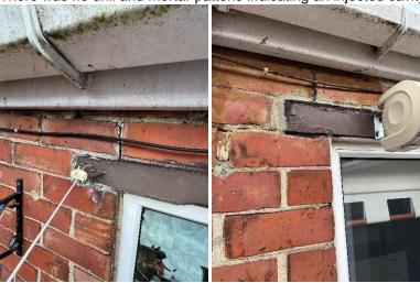
Although considered minor due to the limited loading of 3 course of brick. The masonry has diagonal above the window opening. Diagonal cracking can indicate lintel deflection or structural movement. A lintel supports the masonry above an opening such as a door or window.
