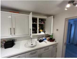
Location of gas meter
