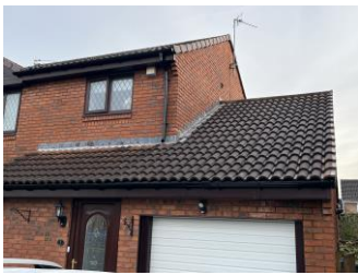
Mono pitched roof over garage
