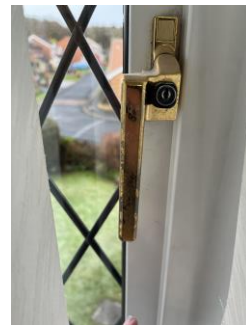
Corrosion on handle
