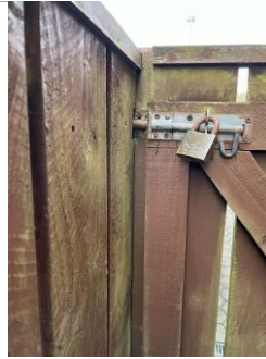
Personnel gate does not close correctly
