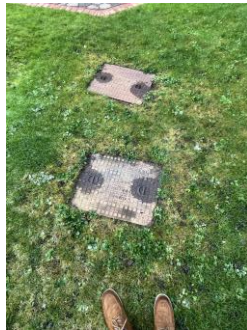
Manholes to rear
