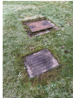
Manholes to front
