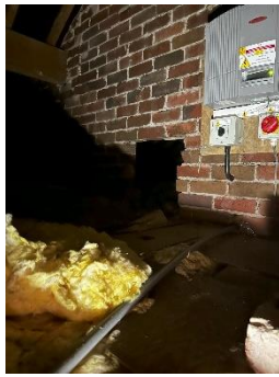
Access to central loft space
