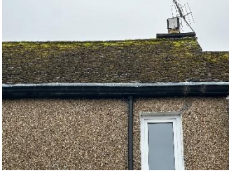
Deflected ridge line
