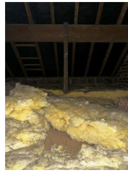
Displace Insulation
