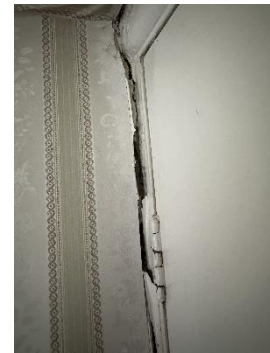
Structural movement
