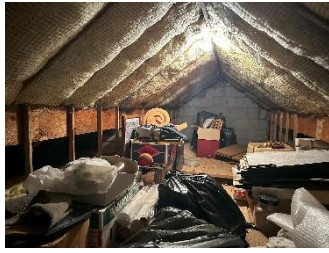
Insulation between rafters and central boarded walk way
