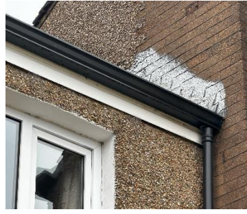
Paint/flash band repair
