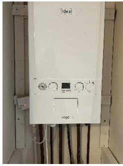
Pic2: boiler installation
