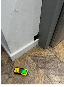
Pic1: small access hole to stop tap
