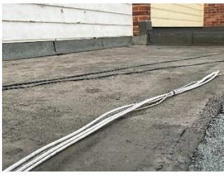
Pic1: Single storey flat roof
