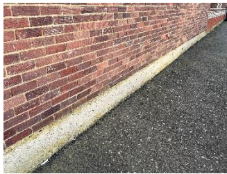
Pic2: Area to l/side of door rebuilt in brickwork
