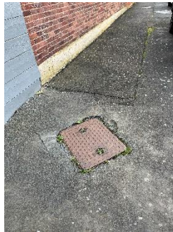
Pic2: Manhole cover front
