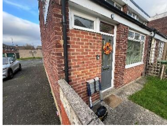
Pic2: Area to l/side of door rebuilt in brickwork
