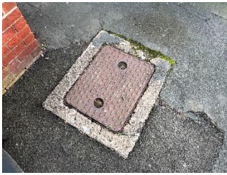
Pic1: Manhole cover rear
