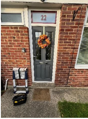
Pic1: Front Access door
