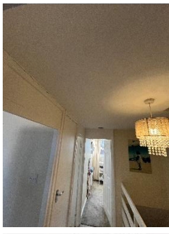
Pic1: Hallway ceiling
