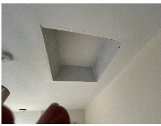
Pic1: Sealed loft hatch
