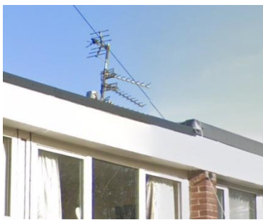
Pic1: View of gas flue terminal
