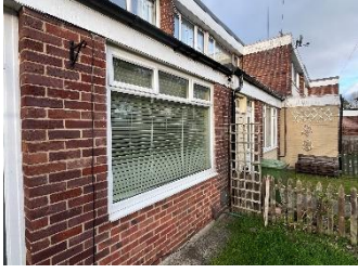
Pic1: Area under window rebuilt in brickwork
