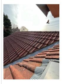
The valley pointing was cracked and missing to the valley roof tile edge line, this is a relatively routine maintenance issue of wet roof applications. Should any damp patches appear inside the roof in the future, then the mortar will need to be checked and replaced to ensure the roof is watertight.
