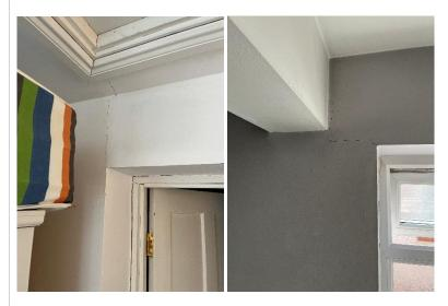
There was plaster cracking to the main bedroom and bathroom walls. The plaster work has also de-bonded from the masonry wall. The plaster should be removed to determine if the cracks are also present to the masonry wall. Structural cracks should be assessed by a Structural Engineer.
