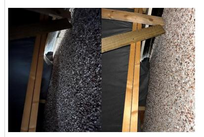
The original gable wall continues between the house and extension, voids are evident at this junction and should be remediated to event insect and moisture ingress
