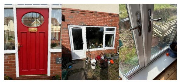
It is advisable to install a door deflector to the bottom rail of the door. A deflector projects rainwater away from the threshold, which helps to reduce the door casing ends from becoming saturated and leading to timber decay.
