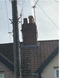
The chimney structure is leaning, this is not unusual for the age of the property. The reason for a leaning chimney stack is from expansion and eroded mortar joints. When the surface of the chimney stack is exposed to the prevailing wind, constant wetting can result in the expansion of
