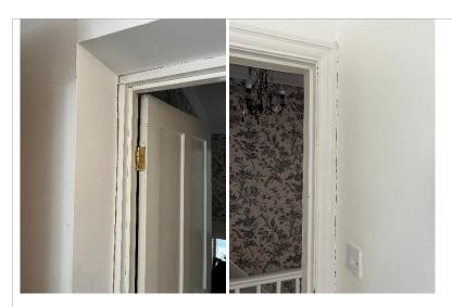
An opening had been formed and altered within the property. Checks should be made to ensure the alteration has been authorised by building control.
