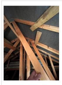
Elements of the diagonal bracing may have also been missed from the construction. The timber bracing provides rigidity to the truss roof structure. A competent person (Truss manufacturer) will be able to determine if an additional timber bracing should be installed.
