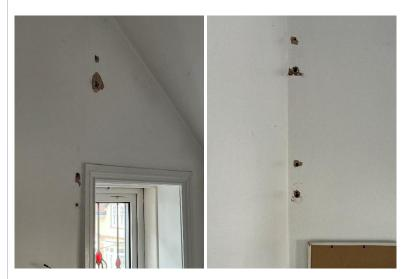
There were several holes to the plaster and partition walls. The holes may be filled with a back board and filled and sanded over.
