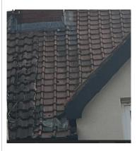
The roof covering tile is a different profile to the neighbouring property. There did not appear to be any damp or water ingress staining internally, however I would recommend the party line upstand is checked by a competent roofing contractor to ensure the installation is in accordance with the manufacturer's guidance and a watertight joint has been provided.
