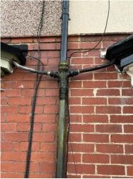
The rainwater downspout joint has a vegetation build up on the joint line which can indicate a defective seal, which is a relatively common maintenance issue. A leaking rainwater downspout over time can saturate/damage the masonry face during cold weather. The vegetation should be
