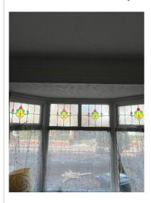
The top openers have dropped and require adjustment as the opener is catching the frame. Openers that do not close into the frame rebate correctly can damage the opener hinge, double glazed unit, and the window frame.
