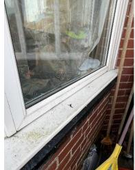
The window frame has external glazing beading which is no longer used in a modern window design. The external beading and double-glazed units can be removed externally. It is advisable to make enquires with the proposed property insurance company, as external glazed beading may be an exclusion from an insurance policy. I would recommend replacing the window frames for property security.
