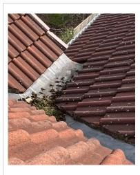
Moss and algae are beginning to form in the valleys, this is a relatively maintenance issue. However, the roof pitch will need to be cleaned in the future with a suitable moss and algae treatment. Moss can hold water, and when frozen can damage the surface of the roof pitch covering over time. Moss can also reduce ventilation which can increase condensation within the roof space.
