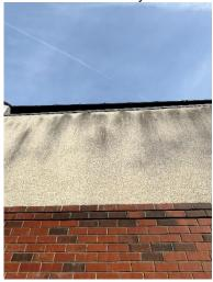
The render below the gutter joint is water stained. The gutter joints should be checked as masonry saturation can damage the mortar pointing, masonry face and can lead to internal damp.
