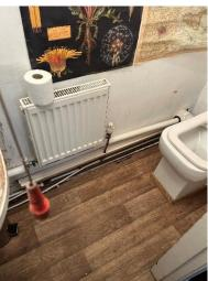
The ground floor WC requires remedial works, the whb is insecure and will need removing and reinstalling with suitable fixings, pipework is exposed and should be suitably encased to prevent damage.
