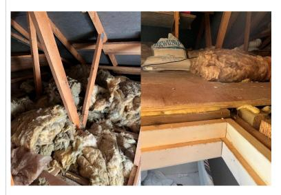
The insulation has been disturbed and requires relaying/replacing to ensure condensation and mould spores do not occur to the warm room ceiling below. The insulation depth should be at least 270mm.
