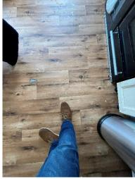
The kitchen floor covering is damaged, it appears the floor covering has been installed incorrectly and without a suitable base. There are also indentations in the floor that should be level to prevent a trip hazard and damage to the floor covering.
