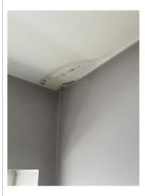
Mould and water staining are visible to the bathroom ceiling, which is adjacent to the hidden box guttering, The guttering will need investigating to check the gutter line and install. The ceiling may also need a water stain block repair and redecoration.
