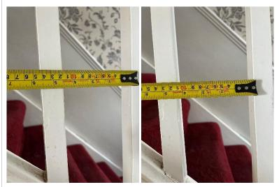
The existing period balustrade and handrail are not to the current building regulation and may pose as a health and safety risk due to a large gap between spindles. The current gap between spindles is a maximum of 115mm.
