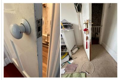
The latch mechanism has also failed in several doors. All doors within the property should be
