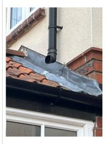
The downspout shoe is installed at a height that will not allow rainwater to expel onto the below roof line as required, an incorrectly fitted shoe can cause rainwater to overshoot the gutter leading to the saturation of masonry below.
