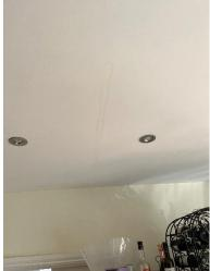
There is water staining to the kitchen ceiling. The water staining should be investigated to ensure there is no water leakage above the ceiling. The ceiling may also need a water stain block repair and redecoration.
