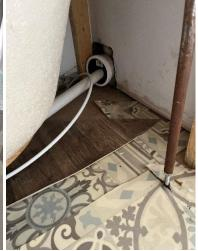
The bath installation is incomplete, and it appears drainage connections are unsuitable, this should be checked by a suitably competent person to prevent further damage.
