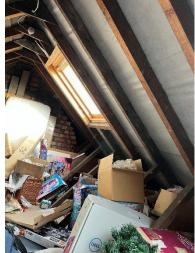
Velux windows have been installed to the rear elevation and the structural design should be checked; the existing roof structure does not appear to be correctly trimmed to take the additional loadings.
