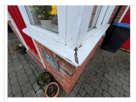
The paintwork to the window has peeled and blistered. The timber requires examining for timber decay and rot and treating/replacement if required. The timber should then be prepared for a new primer, base, and topcoat paint application. It is recommended the external decoration is recoated on a five-to-seven-year cycle.
