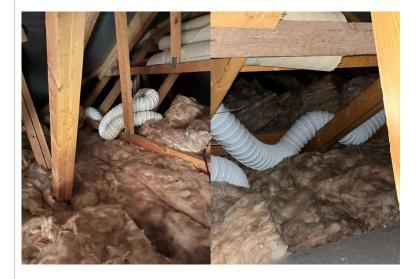
The extractor ducting within the roof space is incorrectly laid which will reduce the unit extraction flow rate. The ducting should be altered to ensure a vertical/horizontal line from the unit to the roof discharge point.
