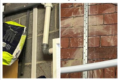
The metal wall plate straps have not been fixed to the masonry during the property construction. The wall plate straps function, is to provide an anchor against roof structure uplift or movement. It is advisable to provide fixings as per the wall plate manufacturers guidance.
