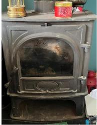
It is unknown if the chimney has been swept and the appliance serviced. If not, both should by checked by a Heating Equipment and Testing Approval Scheme (HETAS) Approved servicing engineer and/or chimney sweep. Your Legal Advisers should make enquires on annual inspection/service records.
