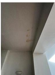
Staining and damage is visible where the extension meets the existing house rear elevation a common defect when an extension abuts an existing structure and no horizontal cavity trays have been installed at the roof abutment.
