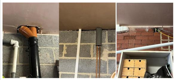
Fire compartmentation has not been maintained through penetrations, where pipes of more than 40mm pass through a fire compartment a suitable fire collar should be installed to maintain its integrity, where smaller penetrations are made then these should be filled with a fir intumescent mastic.
