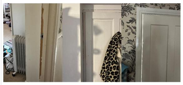
There are period doors within the property that do not close correctly into the door casing. Internal doors that close correctly may slow the passage of fire smoke. It may be a consideration to refit the doors or replace them.
