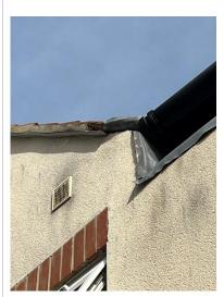
A section of verge pointing was cracked and missing to the roof line edge this is a relatively routine maintenance issue of wet roof applications. Should any damp patches appear inside the roof in the future, the mortar will need to be checked and replaced to ensure the structure is watertight and that the roof pitch tiles cannot be lifted in severe weather.
