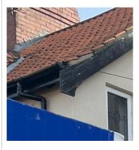
There are sections of the barge board that are decayed and rotten, the extent of which is unknown. Sections of timber rot can be removed and spliced with new timbers, or the length section replaced. Repairing roofline timbers requires scaffold access equipment (which can be costly). I would recommend obtaining estimates of works from competent contractors before the exchange of contracts.
