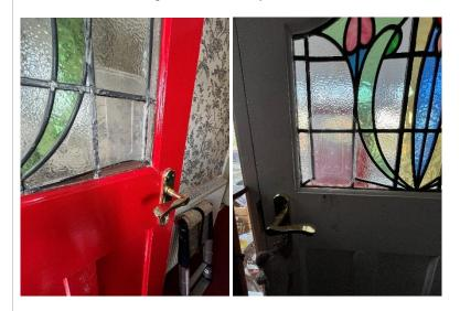
Glazed panel to the front door is damaged/smashed and requires replacing to maintain security requirements.
