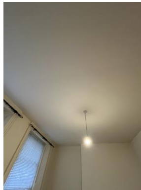
Living room ceiling
