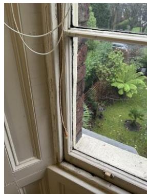
Sash weight ropes cut
