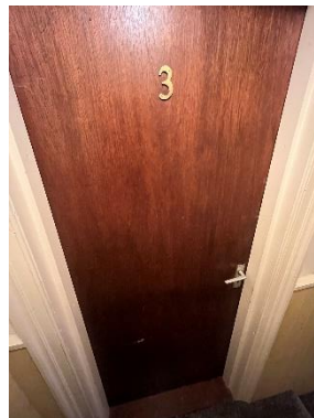
Inside view of front door
