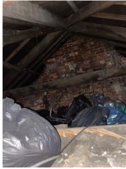
Pic 36: Timber structure
