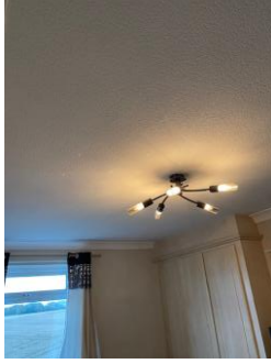
Pic 40: Bedroom ceiling
