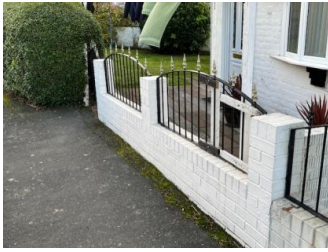
Pic 66: Front gate
