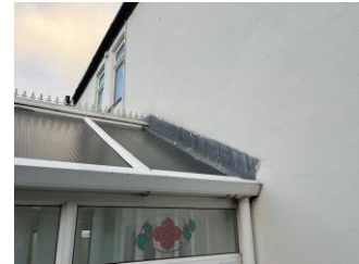
Pic 30: Lead flashing
