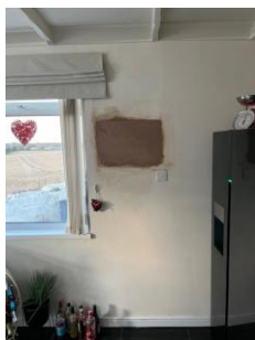
Pic 43: Vent relocated
