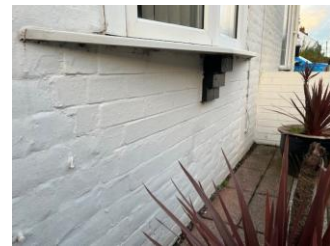
Pic 21 : New brickwork
