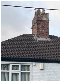
Pic 10: Brickwork pointing
