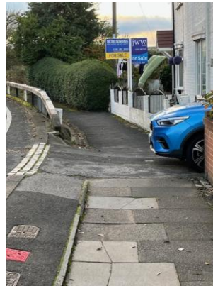
Pic2: Access Pathway
