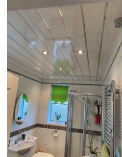
Pic 42: Bathroom ceiling
