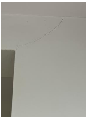
Diagonal cracking
