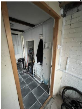
Non fire rated separation
