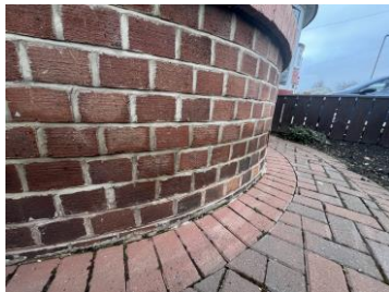
New pointing to bay brick work
