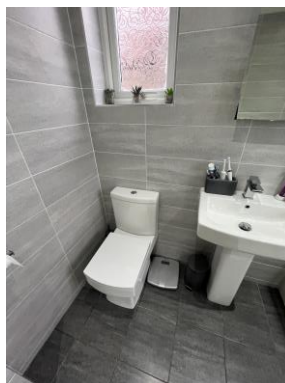
WC and Wash hand basin
