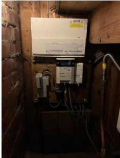
Electric meter and consumer unit
