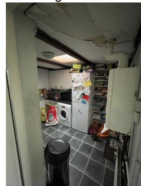
Collapsed ceiling
