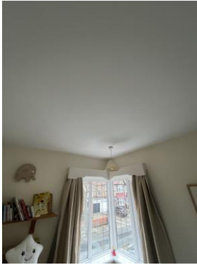
Front bedroom ceiling
