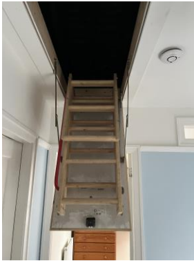
Loft ladder installed for access
