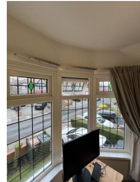
First floor bay window
