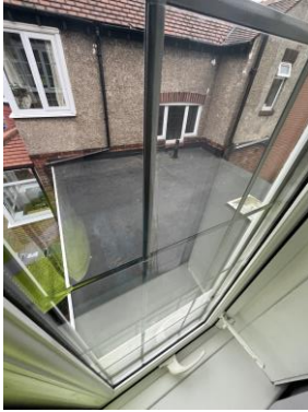
Front corner bedroom window
