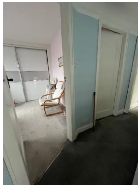
Period skirting and architrave
