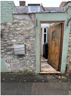
Timber door leading to back lane
