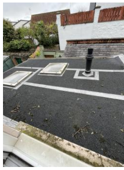
Flat roof penetrations
