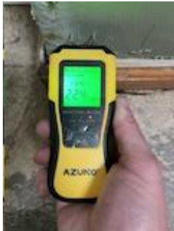
Extension rear wall
