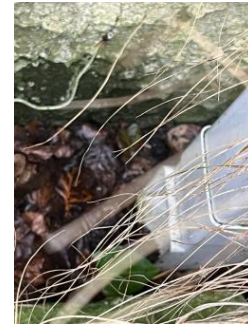
Blocked downspout
