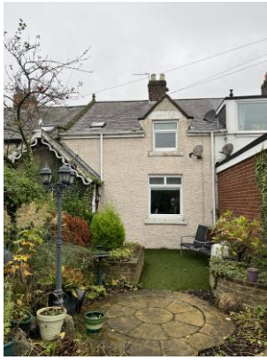
Access through garden
